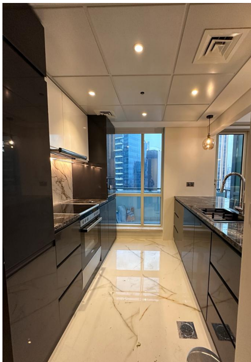
Kitchen renovation project Arabian Ranches, Dubai
