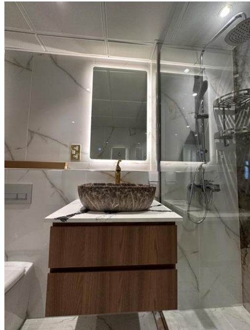
Bathroom renovation Stella Maris Tower, Dubai Marina
